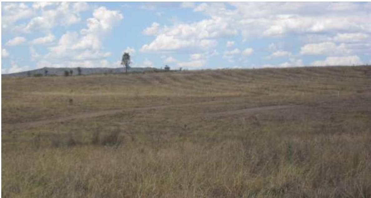
Figure 11: Longwall 3 end line cracks post remediation on the 02/02/2011. The bare patches are where the crack once existed. This image is looking to the north.
