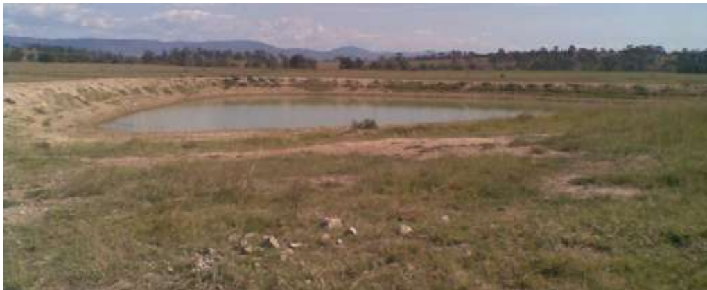
Figure 9: Dam 11 located above the LW6A panel pre undermining on 22/04/2010. The photo was taken looking south west at the centre of the dam wall which is also the lowest point.
