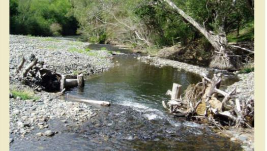
Engineered Log Jam, in this case log step with paired abutment jams. Williams River, NSW
